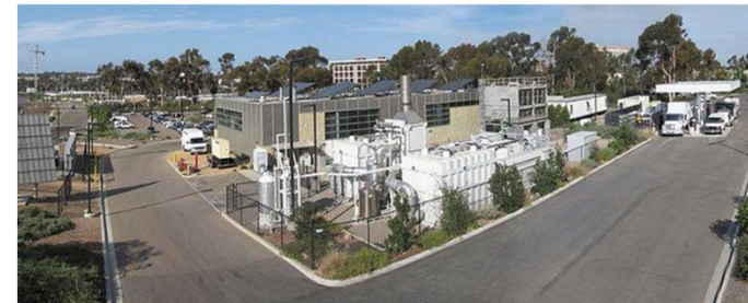
University of California, San Diego (fuel cell installed in microgrid). Photo courtesy of UCSD
