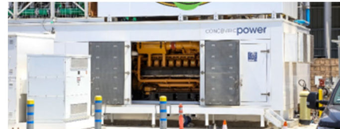
The CHP system currently provides 64% of the facilities power consumption. Photo courtesy of Concentric Power.
