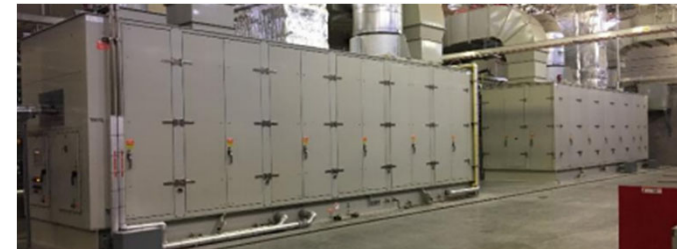
Two Mercury gas turbines. Photo courtesy of Twentynine Palms
