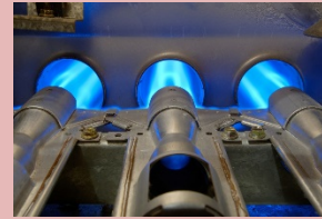
Central Furnace Burner
