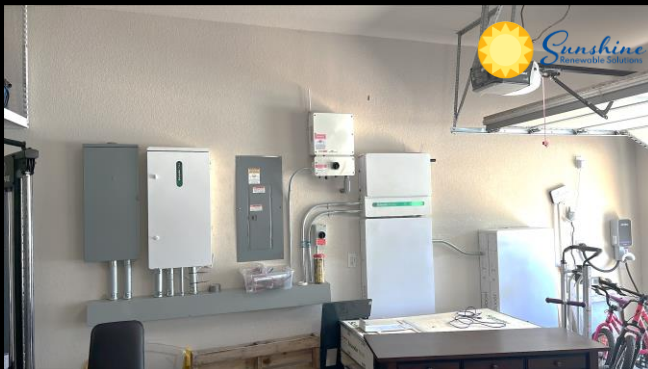
Schneider Pulse Backup Controller, Schneider Inverter, 3 x Schneider Boost, Square D Smart Relays
